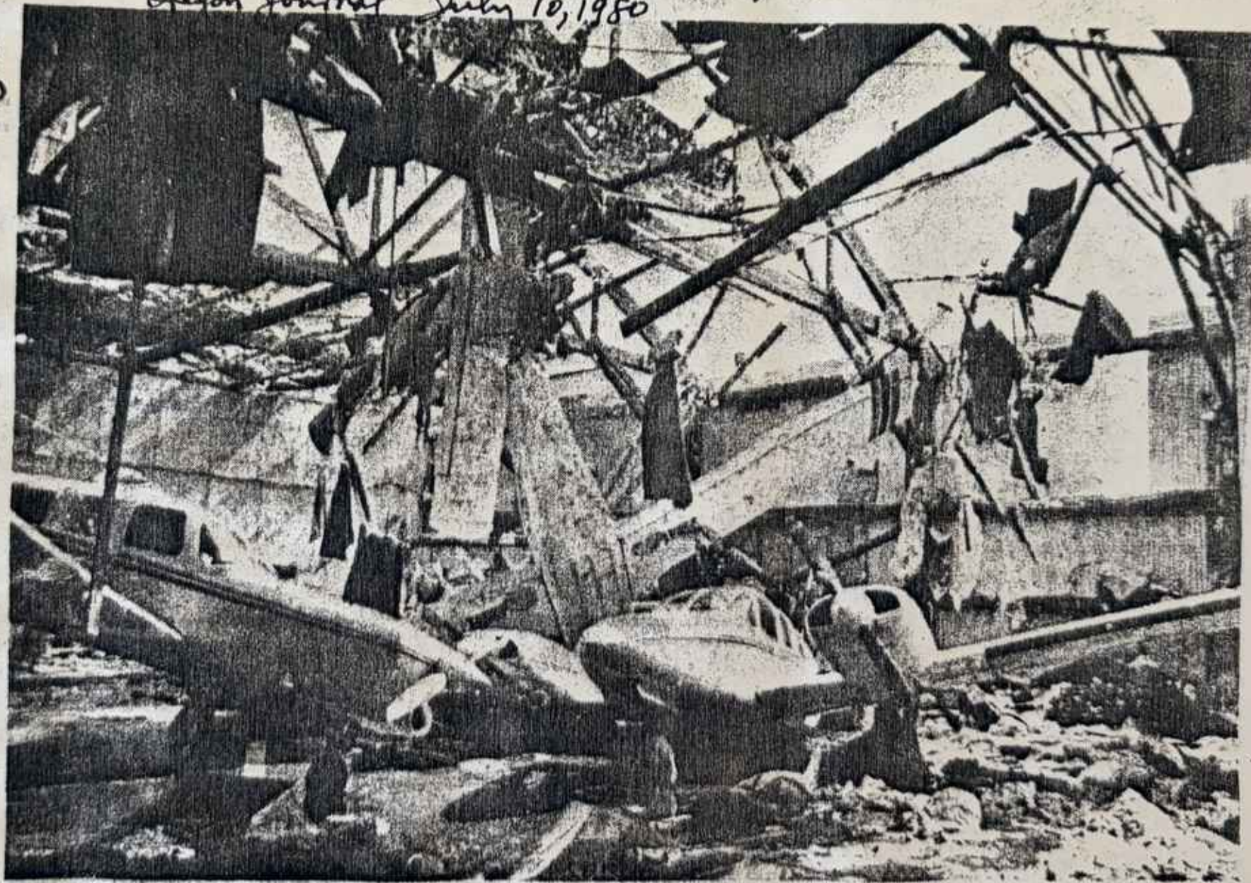
HANGAR DEMOLISHED — Wind of more than 100 mph hit Waterloo, Iowa, causing major damage to Waterloo Municipal Airport. Dozens of private
