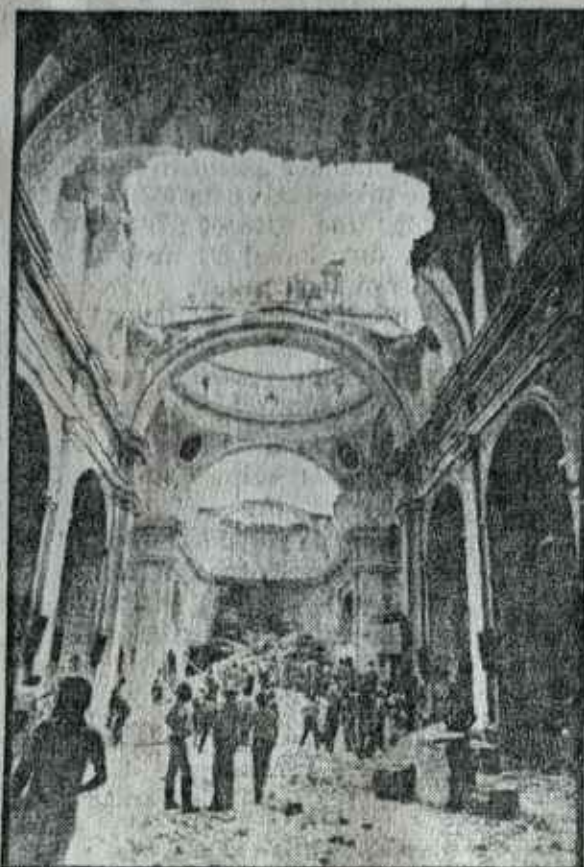
27 died when the roof of Popayan's cathedral collapsed.
